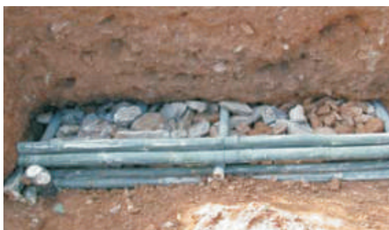
Figure 32: Construction steps of a vegetated bamboo crib wall
