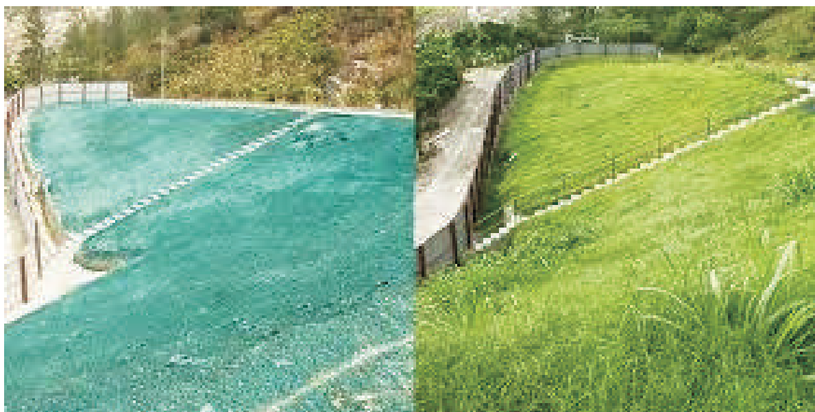
Figure 31: Site Situation at the time of Hydro-seeding and sometime after Hydro-seeding (Bluetgarden)
