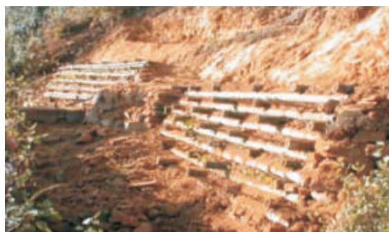
Figure 32: Construction steps of a vegetated bamboo crib wall
