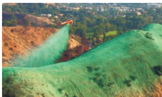
Figure 30: Aerial Hydroseeding (Polymer Innovations)
