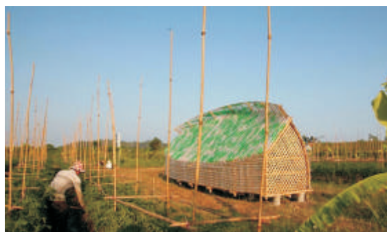
Figure 38: Base of house is made up of concrete
